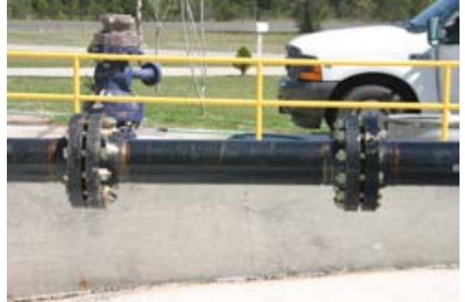
Figure 5: Overview of Replaceable Defect Section
